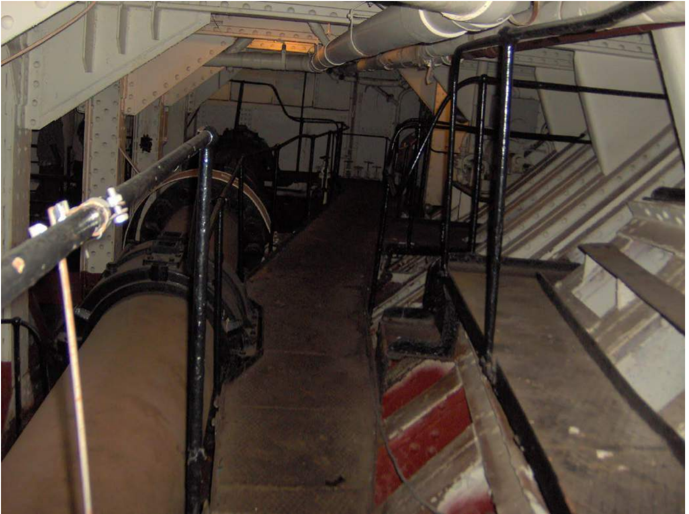
Figure 53 - One of the shaft tunnels - a gloomy place
