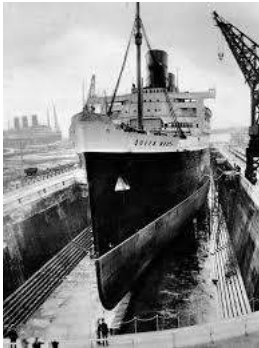
Figure 22 - Not quite enough water in the dock yet...
