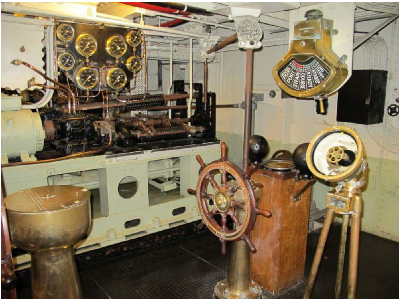
Figure 73 - The Steering Gear Telemotor showing the hand wheel from the after flying bridge
