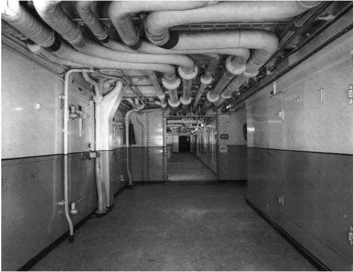
Figure 58 - The Burma Road - Working Alleyway, Port side D Deck
