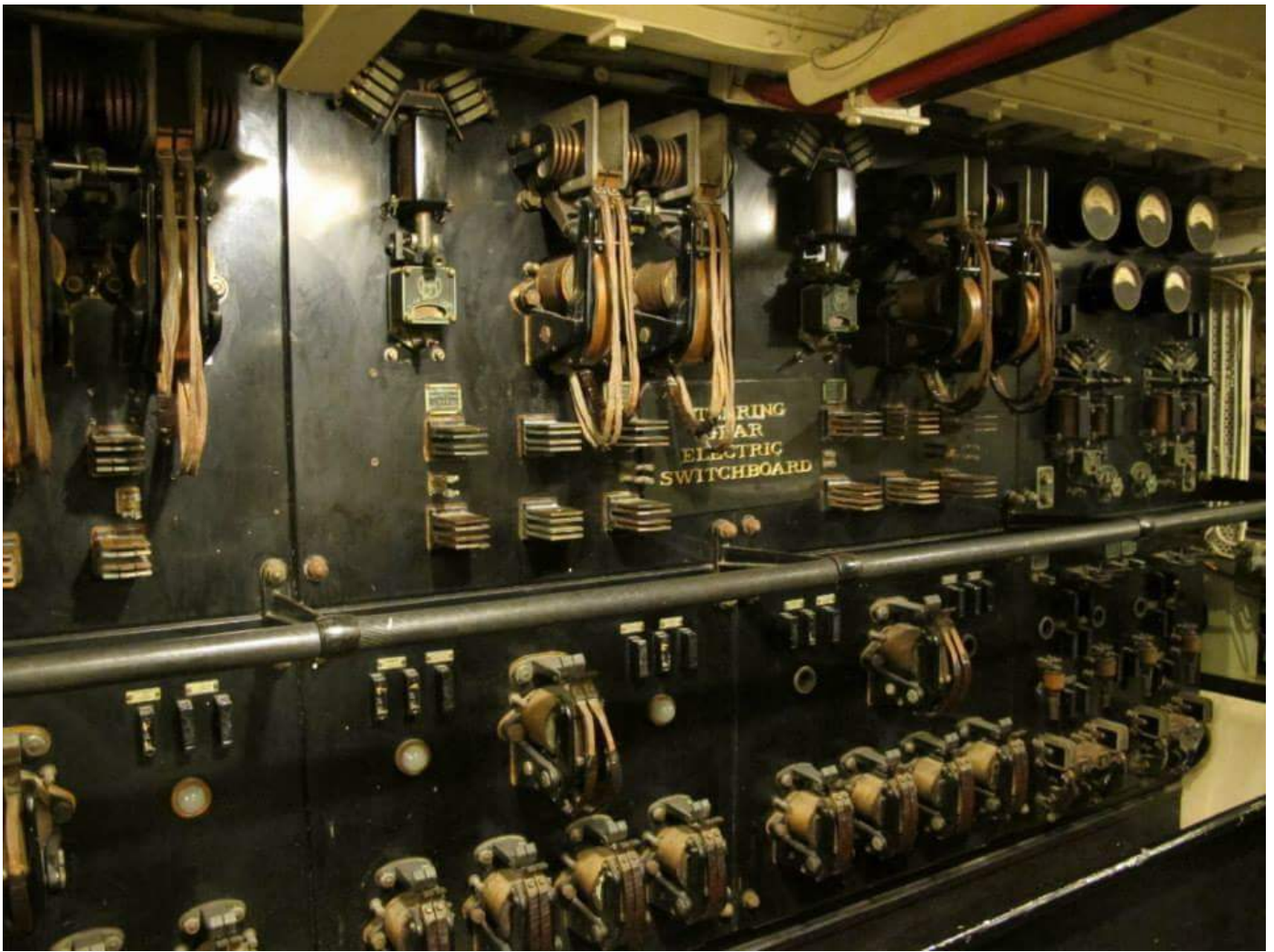
Figure 74 - The Steering Gear Switchboard
