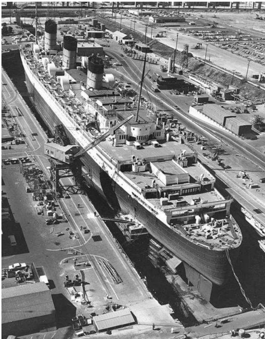
Figure 6 - showing the dry-dock entries in the hull aft above the port outer propeller
